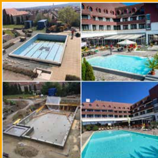
SWIMMING POOL RENOVATION
